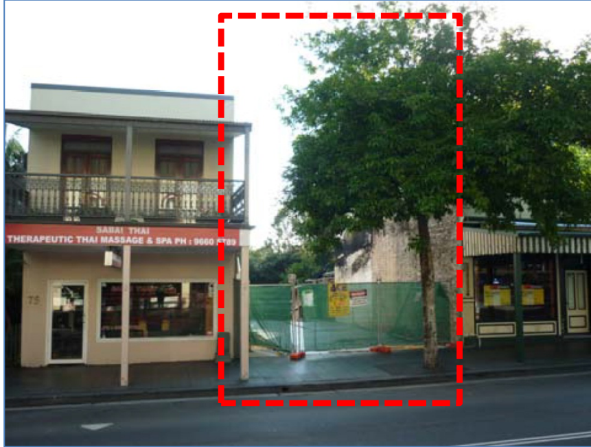
Figure 6: 73 Glebe Point Road Glebe as a vacant site, April 2013
