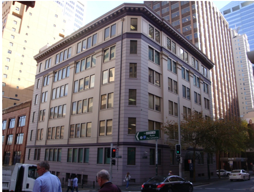
Figure 8: 453 Kent Street Sydney as at May 2014
