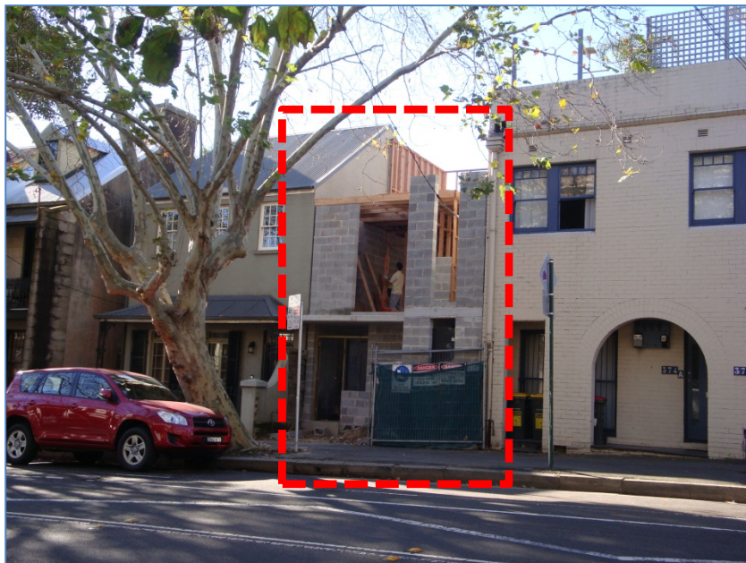
Figure 5: 372 Riley Street, Surry Hills as at June 2014
